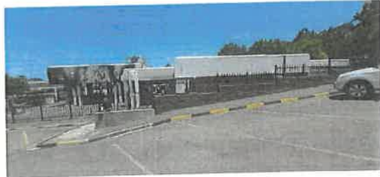
Side elevation of building with only smoke damage
