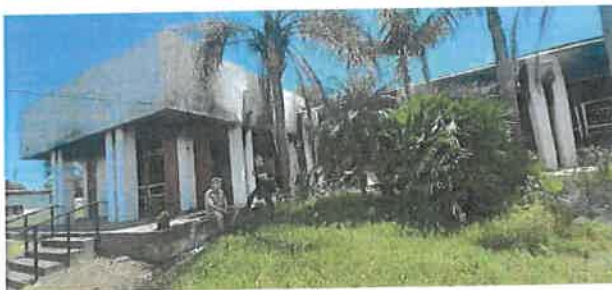
Photo 2.3: Side elevation of building with fire damage visible on the concrete frame.
