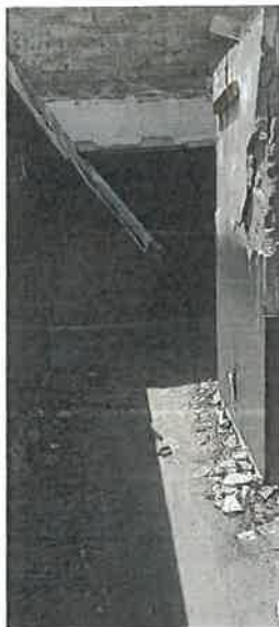
Phase 1 hallway rated 2 roof purlins gone Entrance door was bricked up after the fire
