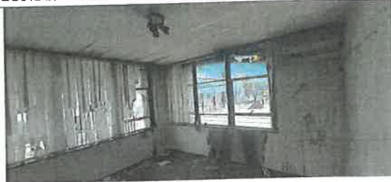
Gerrit Louw's office rated 2
