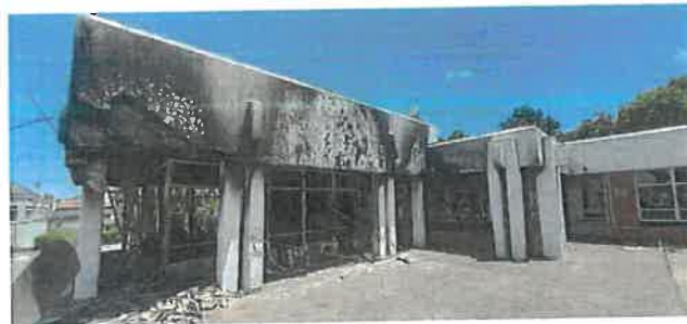
Photo 2.3: Side elevation of building with fire damage visible on the concrete frame.
