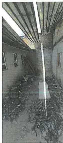
Phase 1 hallway rated 2 roof purlins gone Entrance door was bricked up after the fire
