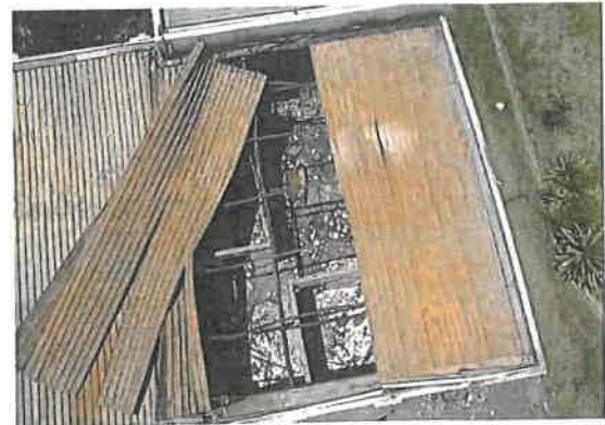
Photo 2.1: Aerial view of Municipal Headquarters building, with roof structure with visible damage Photo 2.2 close up view from above at severely damaged area.
