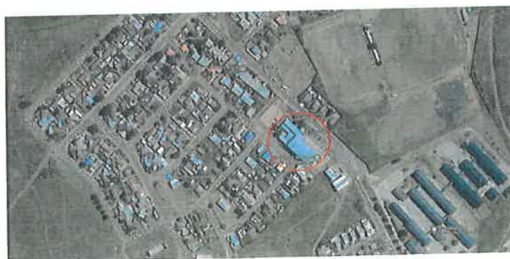
Photo 1.3.2: Thusong Community Centre in the outskirts of town.
