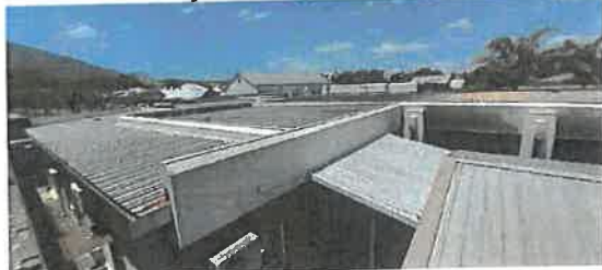
Back view of roof
