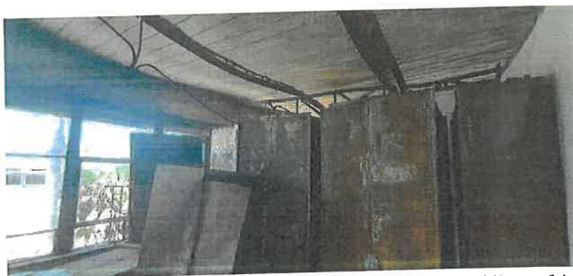
Photo 3.9 & 3.10: Central passage with extensive fire damage visible. Note the filing cabinets in the offices that had lots of documents, that fuelled the fire to be more intense in those areas.
