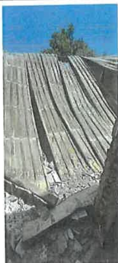
Roof structure destroyed at offices at origin of fire, with records room.
