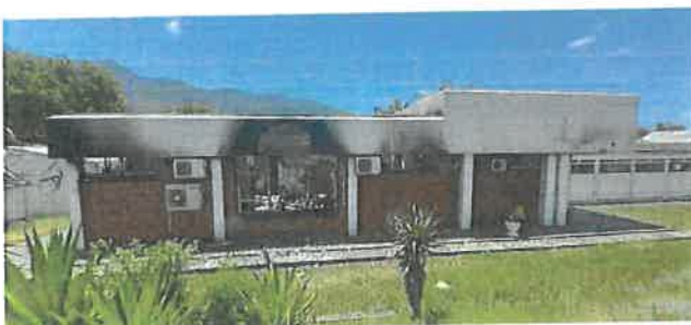
Photo 2.4-2.7: Various elevations of the building with fire damage on the external concrete frame.
