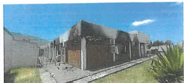
Photo 2.4-2.7: Various elevations of the building with fire damage on the external concrete frame.
