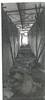
Photo 3.9 & 3.10: Central passage with extensive fire damage visible. Note the filing cabinets in the offices that had lots of documents, that fuelled the fire to be more intense in those areas.
