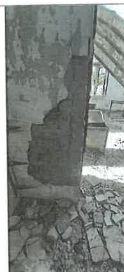
Brick walls with large cracks from fire damage
