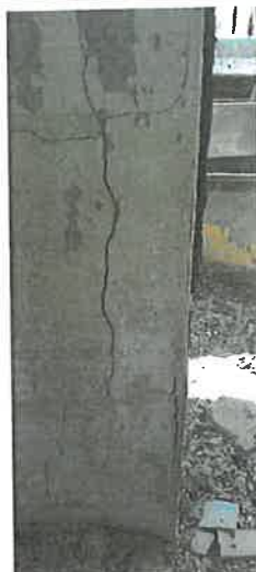
Brick walls with large cracks from fire damage
