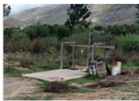
Sewer manholes (82 Houses)
