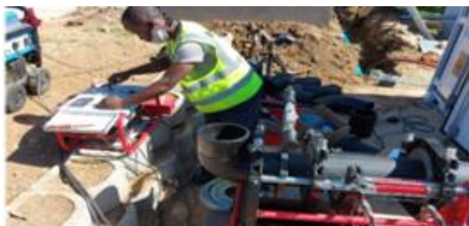
Suurbraak, Upgrade of irrigation pump station
