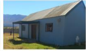
Construction of the Buffeljagsrivier Multi-Purpose Facility
