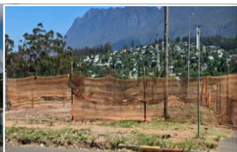
Upgrading of the Railton Pump Station
