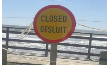
Repair of Kabeljou bank stairs
