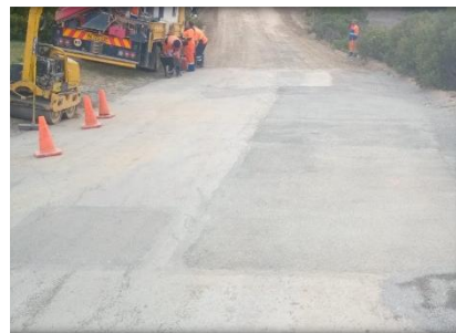
Upgrading of Bontebok Landfill site
