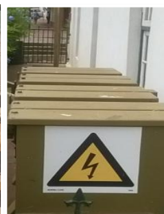
Replacement of Old redundant MV oil
