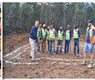
Water pump station
