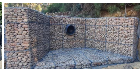
Storm Water Relief Grant
