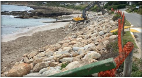
Road bank stabilization
