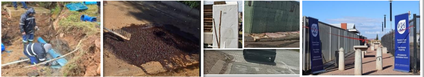
Upgrade Sewerage system
