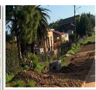
Upgrade, street front sewers
