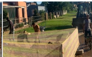
Upgrade, Street Front Sewers Fixing
