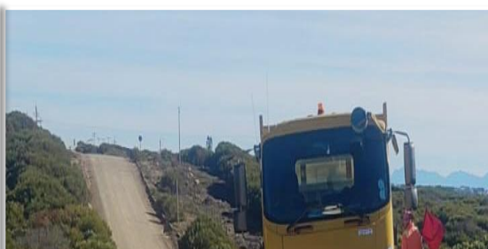
Road Maintenance and cleaning of
