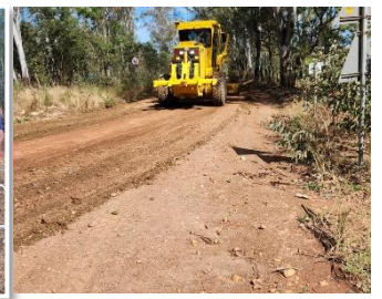
Upgrade Hermitage Road
