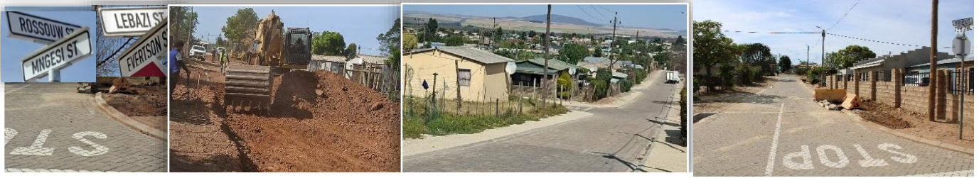
Railton Rising Main
