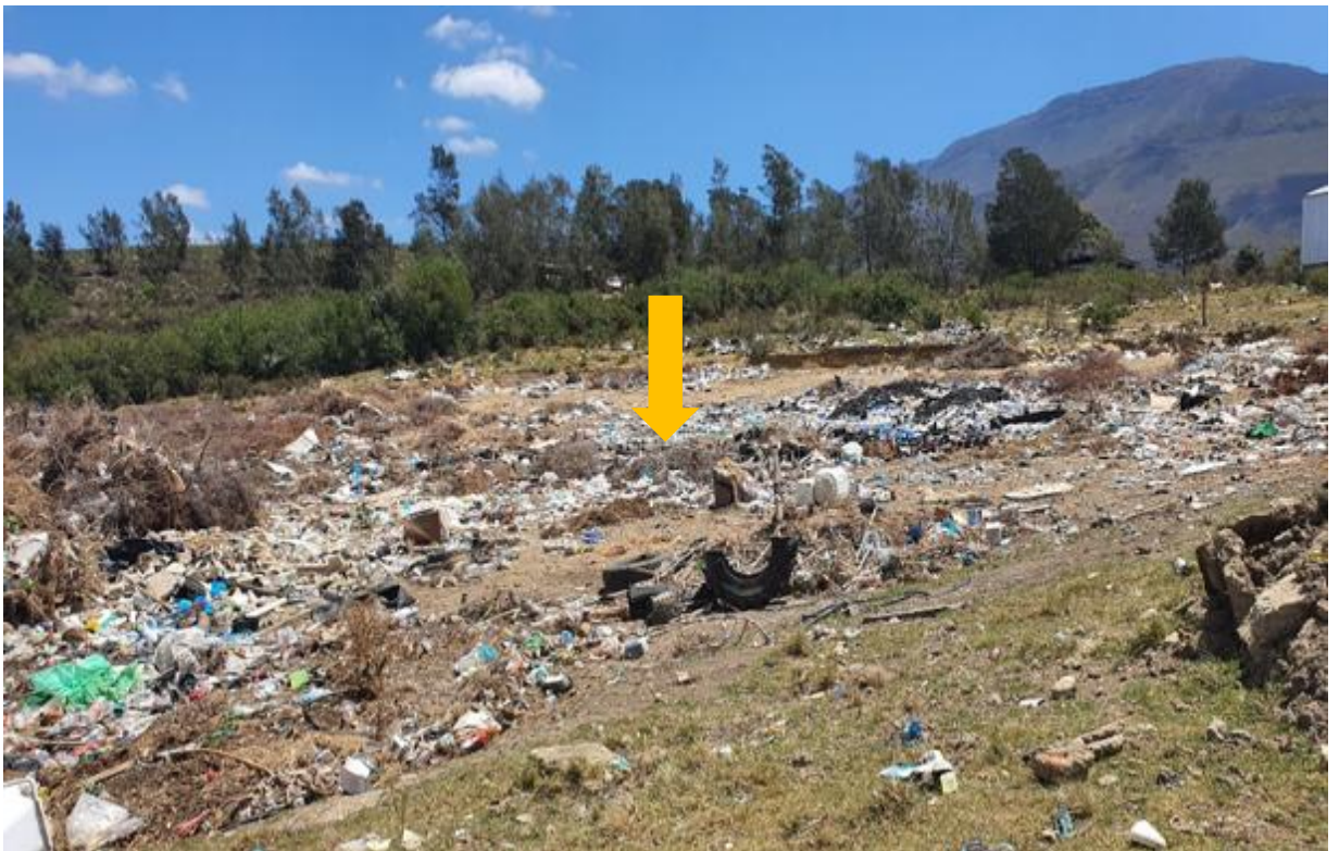
Photo 2: Overview of the Suurbraak Waste Disposal facility - waste is not covered and the facility is not fenced off.
