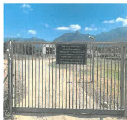
No Access Control Measures Before Entering the Wastewater Plant
