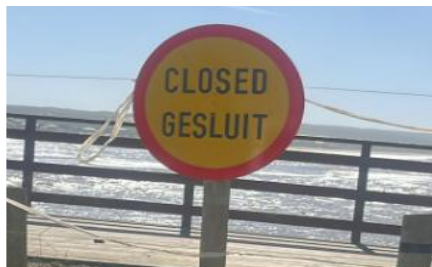
Repair of Kabeljou bank stairs
