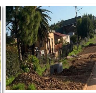
Upgrade, street front sewers
