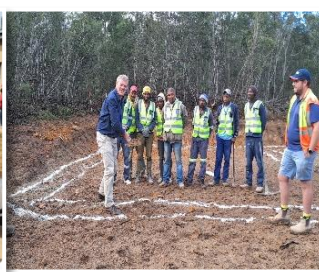
Water pump station
