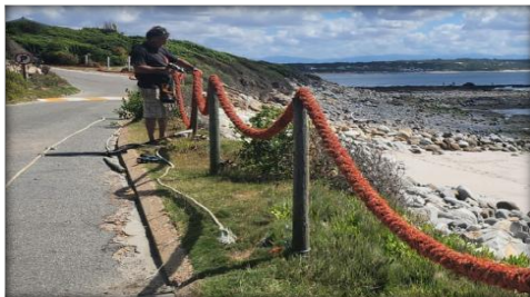
Upgrading of Infanta Slipway
