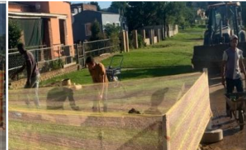
Upgrade, Street Front Sewers Fixing
