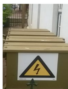
Replacement of Old redundant MV oil
