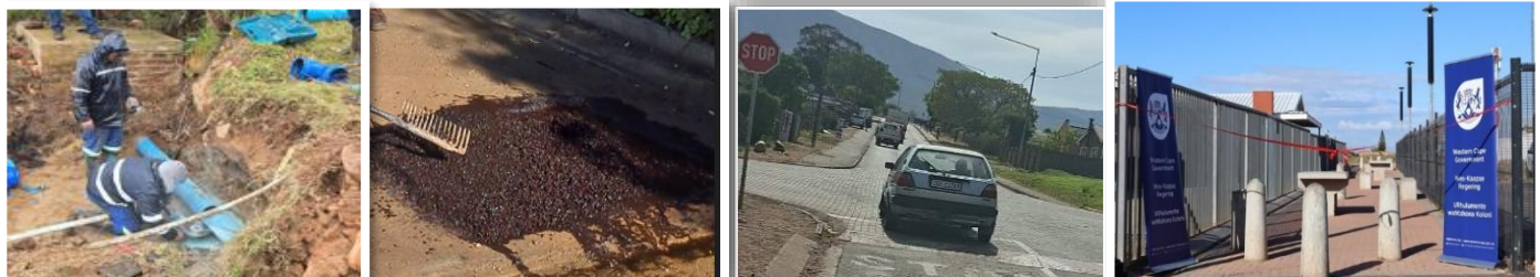
Upgrade Sewerage system
