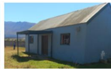
Construction of the Buffeljagsrivier Multi-Purpose Facility
