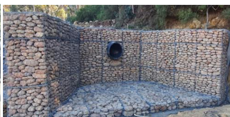
Storm Water Relief Grant
