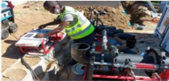
Suurbraak, Upgrade of irrigation pump station
