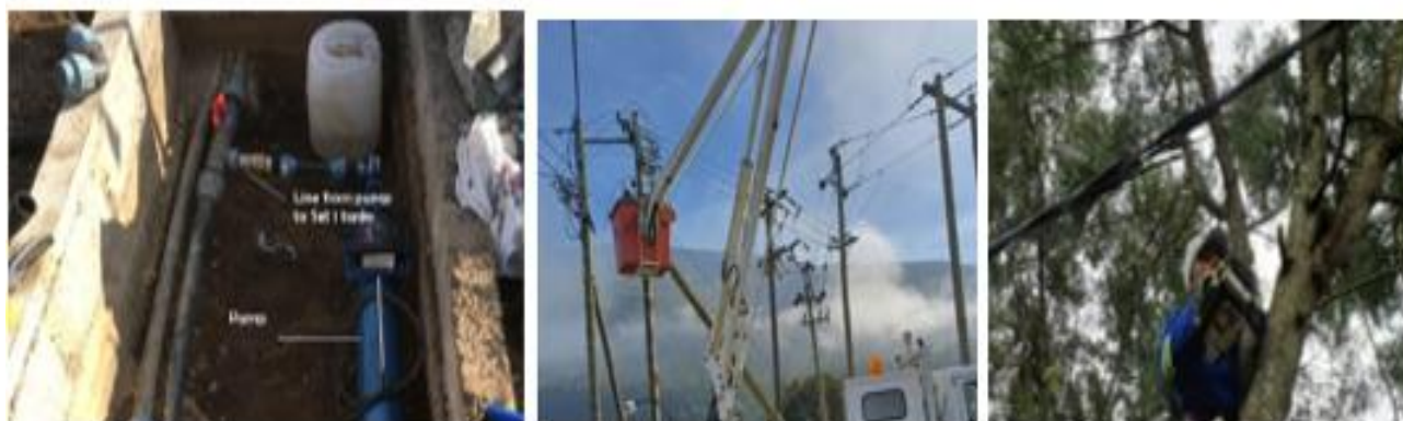
District new reservoir
