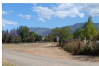
Buffeljagsrivier Housing Project: Construction of houses
