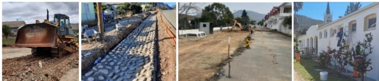
Smitsville Storm water upgrading
