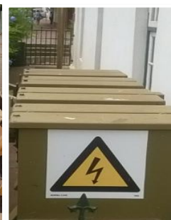
Replacement of Old redundant MV oil
