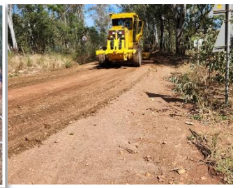
Upgrade Hermitage Road
