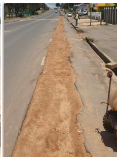
Upgrading of water networks: Railton rising main
