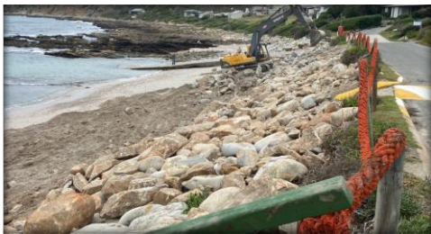
Road bank stabilization
