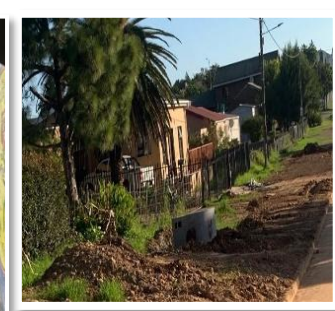
Upgrade, street front sewers
