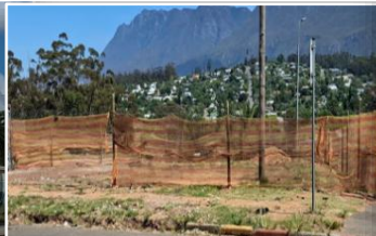
Upgrading of the Railton Pump Station
