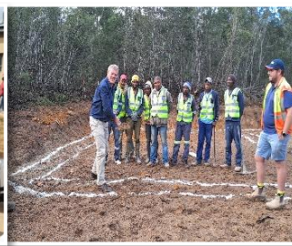
Water pump station
