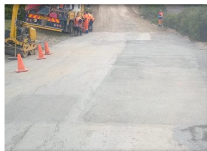
Upgrading of Bontebok Landfill site
