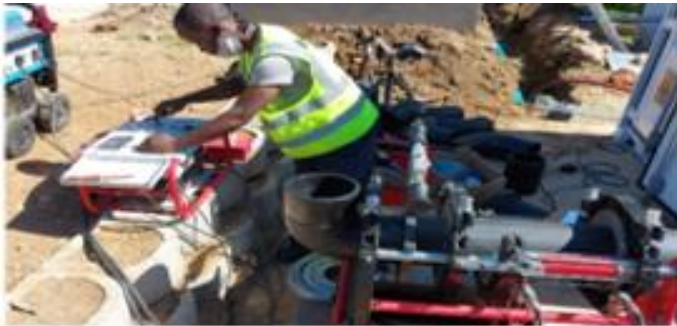
Suurbraak, Upgrade of irrigation pump station
