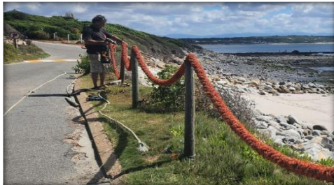
Upgrading of Infanta Slipway
