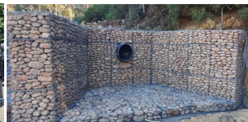
Storm Water Relief Grant
