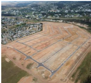
950 Railton Housing Project
