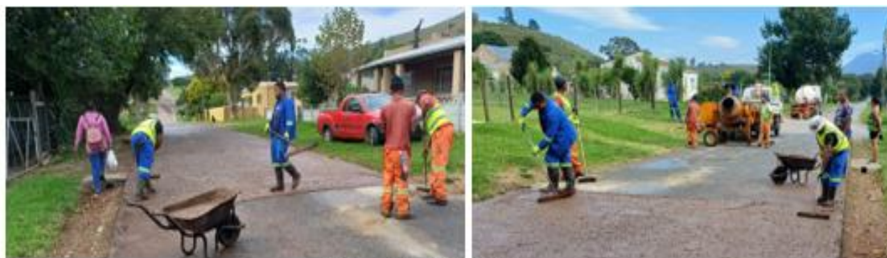
Roads and Storm Water Maintenance
